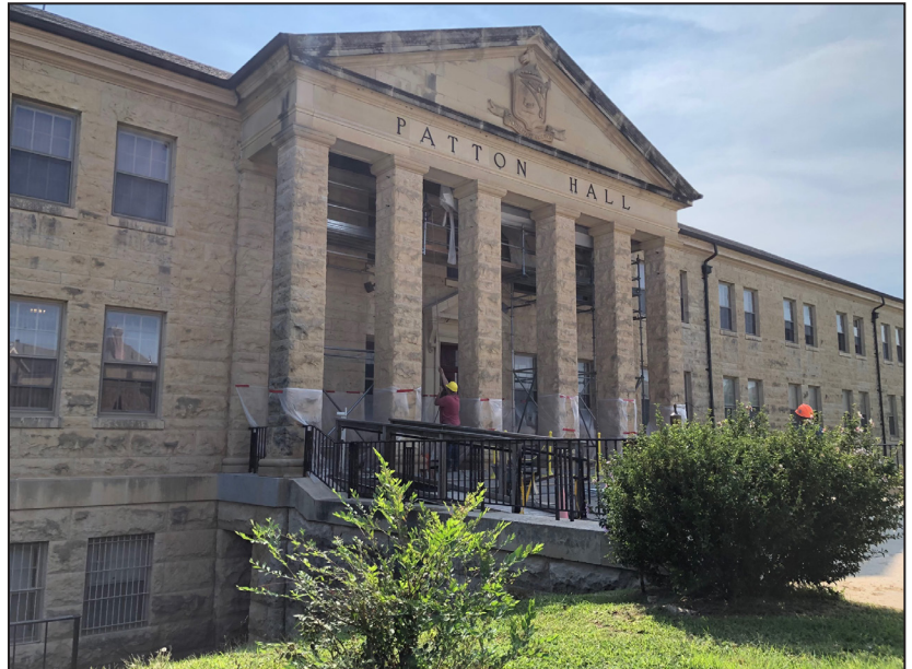
Workers perform repairs on the main entryway ceiling at Patton Hall in Fort Riley, Kansas.
